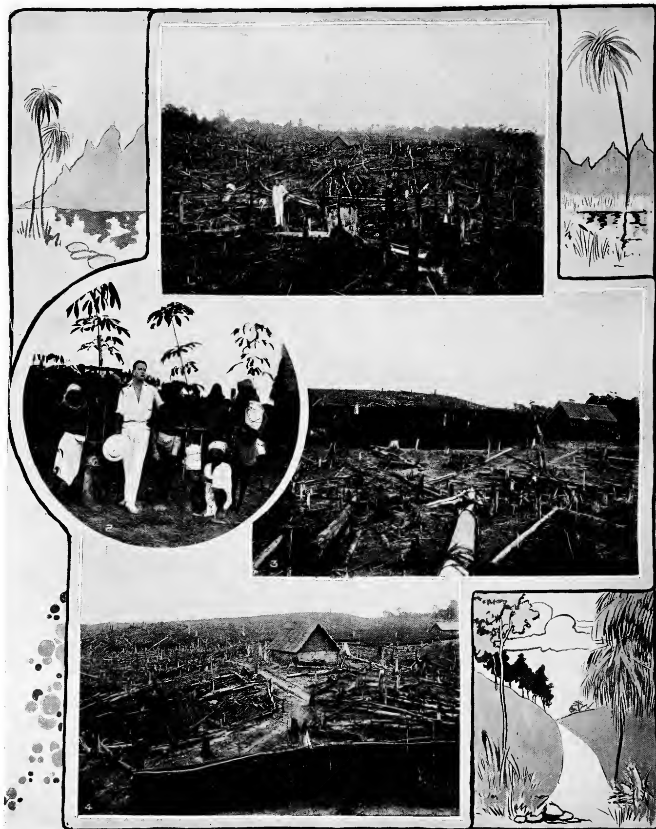
1. GENERAL VIEW OF CLEARING.
