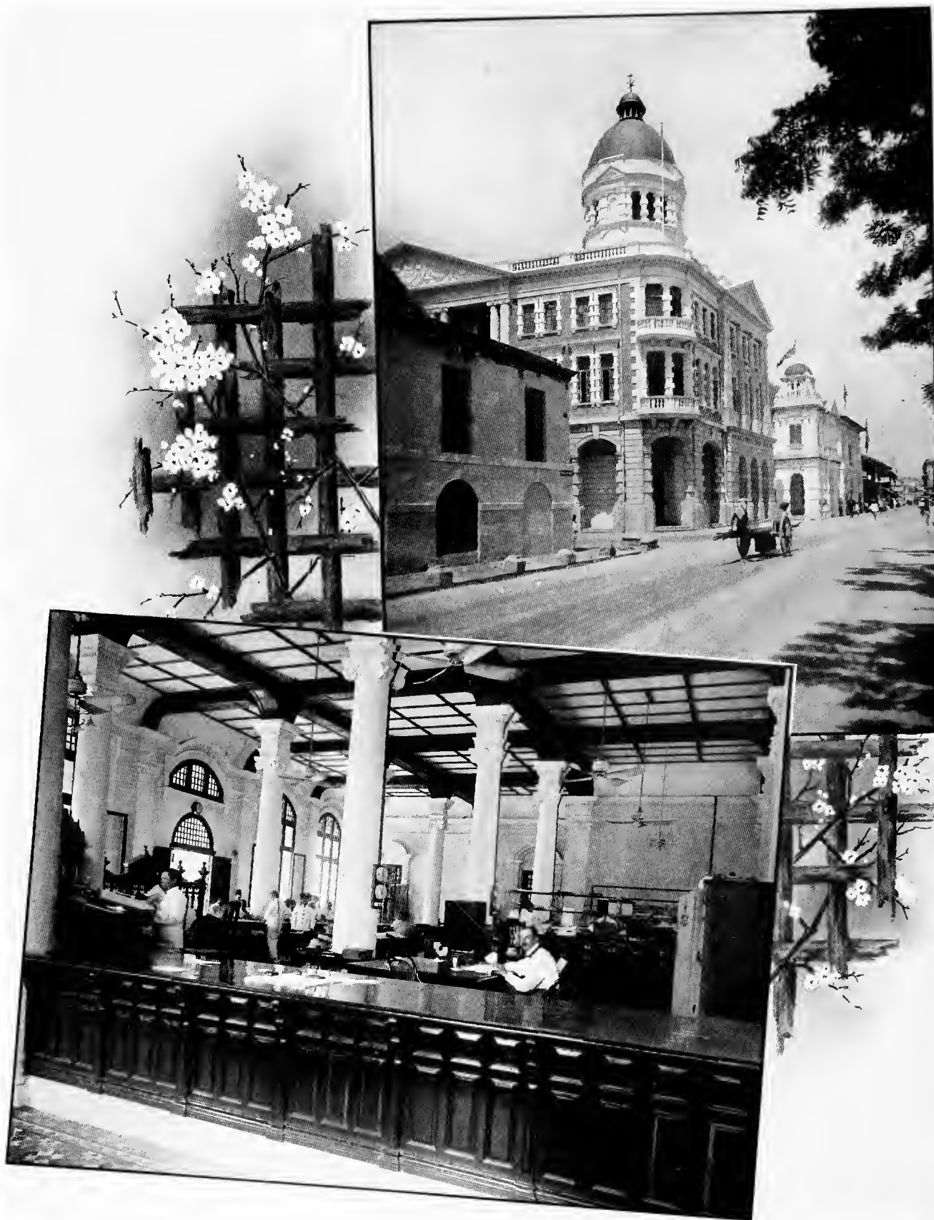
HONGKONG AND SHANGHAI BANKING CORPORATION, LTD., PINANG.
