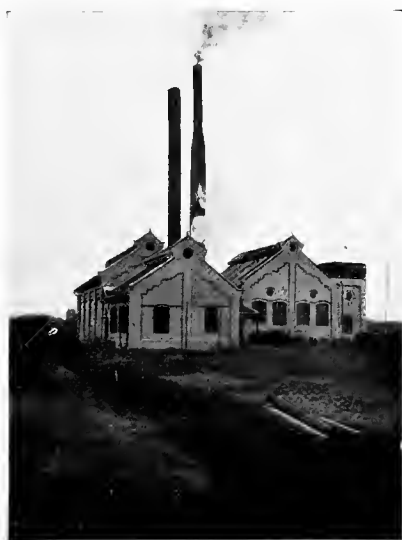
THE ELECTRIC POWER STATION.
